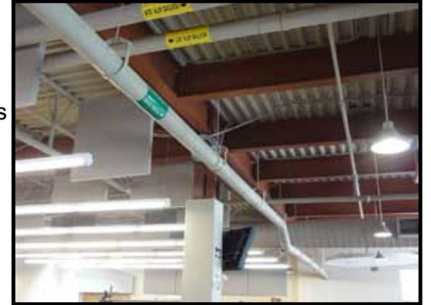
The water is then piped separately for the grey water uses mentioned above, first travelling past an ultraviolet light to kill any bacteria in case someone was to accidentally drink the water.
