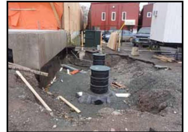
In the parking lot there is a special “Stormceptor” connected to the catchment drain. This traps and then prevents sediment and oil from flowing from the parking lot into Brierly Brook. The Stormceptor is buried in the ground directly behind the library under the laneway.
