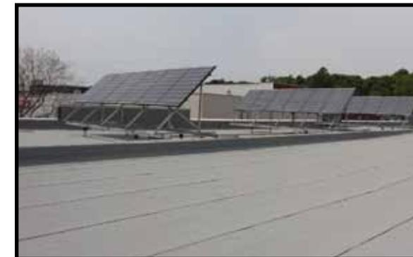
The second solar system energizes the hot water heating system. These two arrays are located on the north section of the roof and water is pumped through the vacuum tubes. Rebates are available for these hot water systems.
